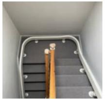
The neat and clean looking track fits securely to the staircase. Each track is built to fit each individual staircase.
